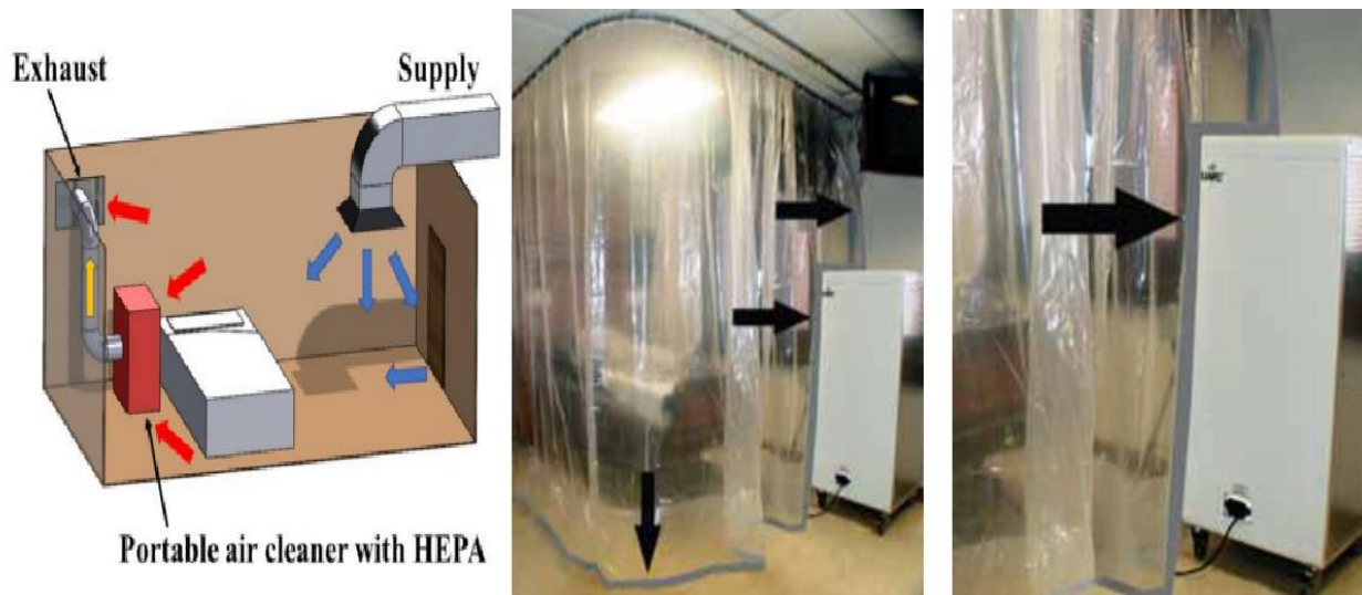
Figure 23: If windows cannot be used and the recirculation mode of the ACMV cannot be terminated, use portable air cleaners with HEPA filters with an exhaust installed to the outside after turning off the ACMV. The air cleaners should be placed close to the head of the patient. See reference 2 for details.
