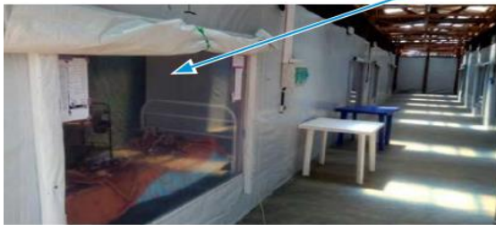
Figure 27: While closed doors are important, it is also vital to be able to observe the patient closely. Transparent observation windows or doors are therefore required. See reference 5 for details.
