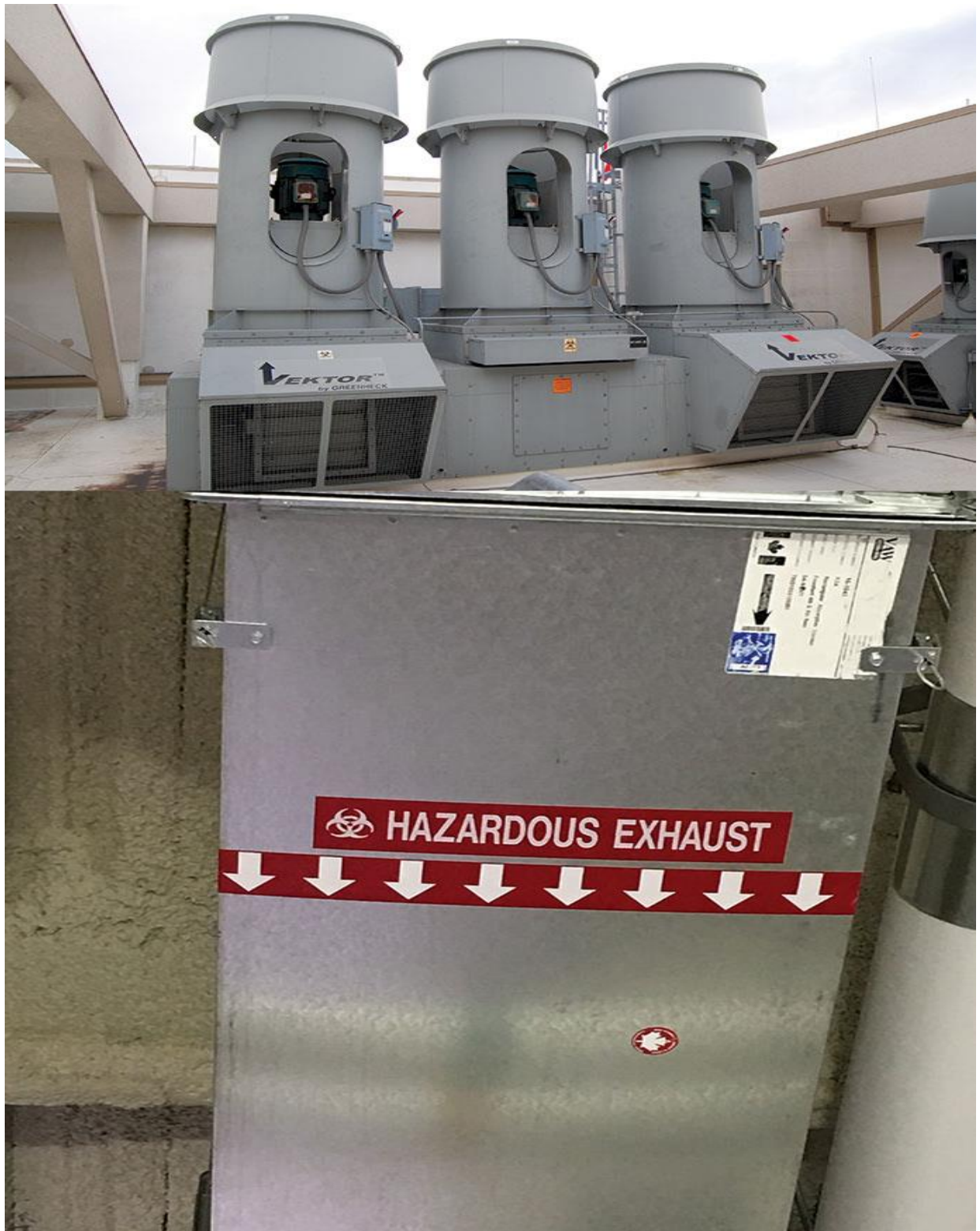
Figure 25: The exhaust fan should be located outdoors and placed as far away from intakes and public areas as practical with discharge above the roof. If serving isolation rooms, such exhausts should be labelled as hazardous. See reference 3 for details.
