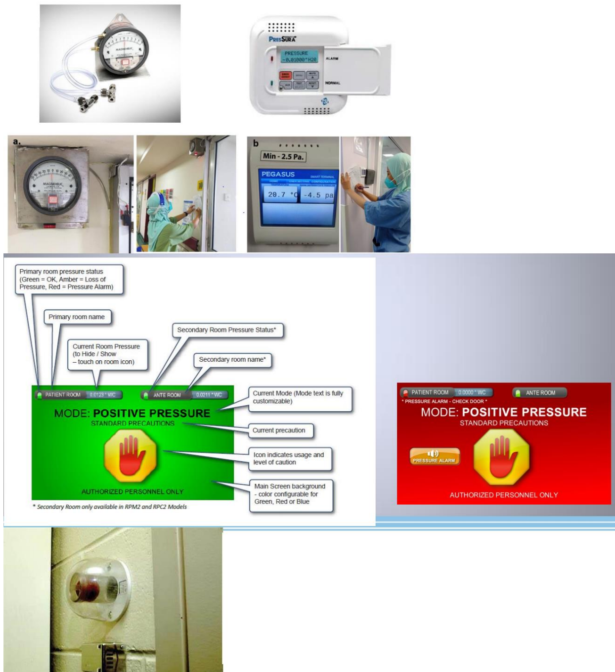
Figure 31: Pressure monitors are mandatory for negative pressure rooms in order to ensure the absence of leakage of air. Smoke test kits, portable manometers and the paper test can also be utilized. While some of the above pictures depict positive pressure mode, actually, negative pressure is required in order to isolate patients with High Consequence Infectious Diseases. See references 2, 6 and 7 for details.
