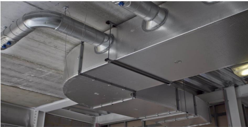
Figure 22: Ducted air-conditioning and mechanical ventilation (ACMV) systems with recirculation mode. If windows cannot be opened and such ACMV are in use, set the system to be mixed with 100% outdoor air (but ensure good control of humidity is maintained) and terminate air return mode. It is preferable to install HEPA filters on the air return duct. See reference 2 for details.
